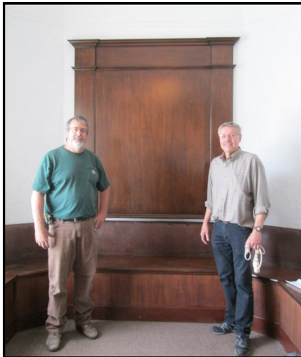
donor appreciation wall on installation day
