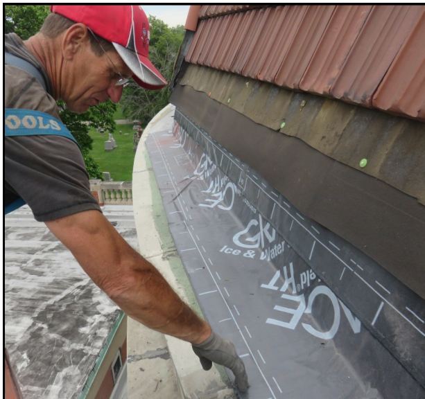
gutter system, membrane
