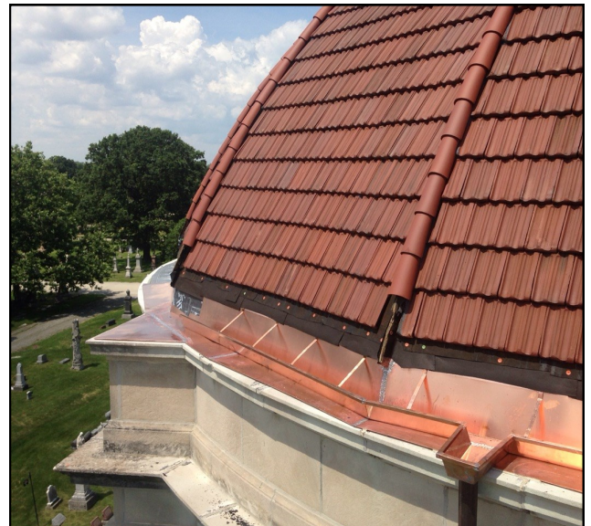
gutter system, new copper
