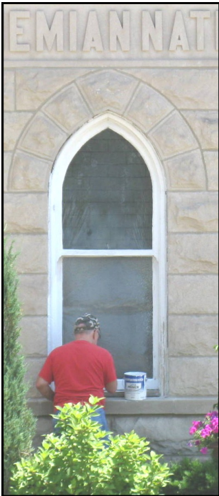
Jerry Gaydusek paints a gatehouse window. (photo by Chuck Michalek)
