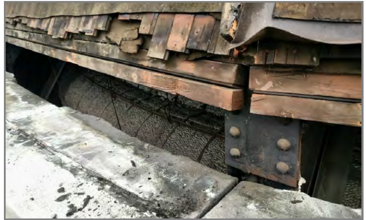
After removing the decaying materials (above), Knickerbocker installed new weatherproofing membrane and added 24-ounce copper features, including flashing, drip edges and downspout scupper boxes. Photos courtesy of Knickerbocker Roofing and Paving Co.
