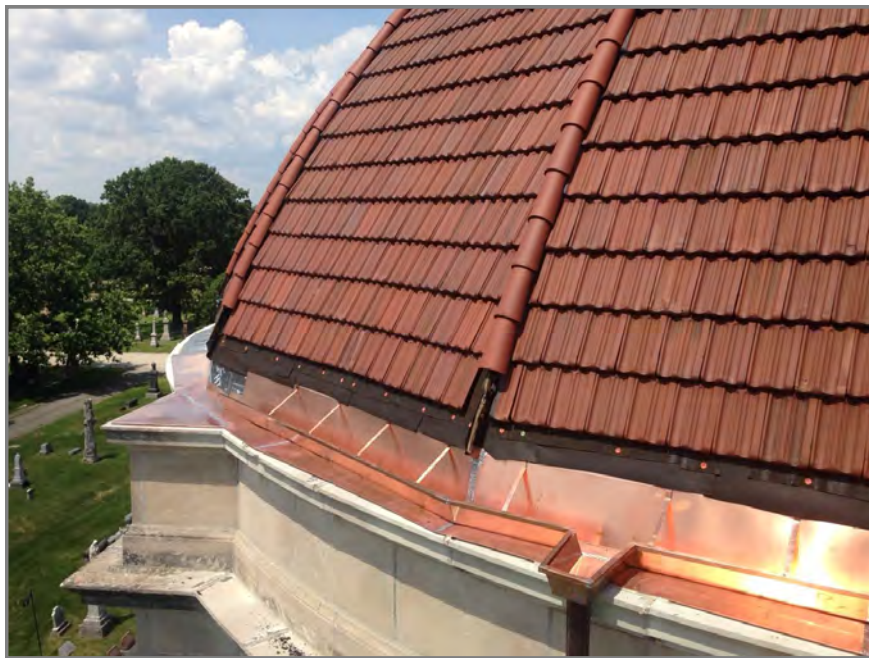
After removing the decaying materials (above), Knickerbocker installed new weatherproofing membrane and added 24-ounce copper features, including flashing, drip edges and downspout scupper boxes. Photos courtesy of Knickerbocker Roofing and Paving Co.
