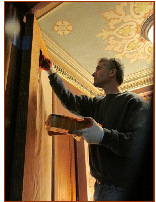
Tony Kartsonas working on the interior doors of the crematorium/columbarium vestibule
